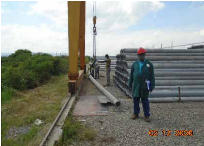
Figure 4: FAT for concrete poles
