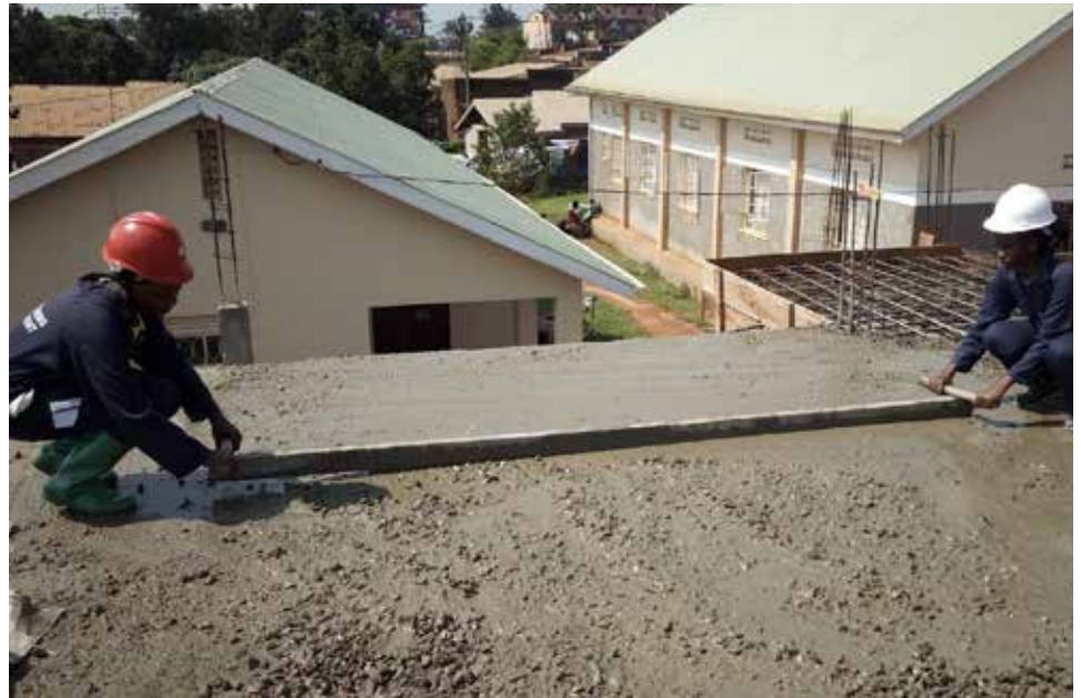
Figure 1: Graduate interns on site levelling concrete
