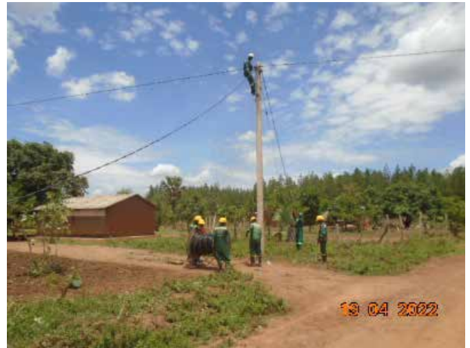
Figure 7: Ongoing works by Haso Engineers
