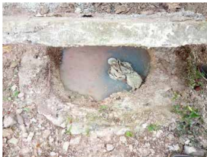
Figure 1: Showing the underground pit
