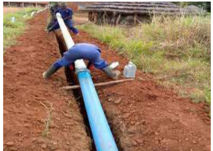
Figure 4: Pipe laying of Lemo-PTC transmission mains
